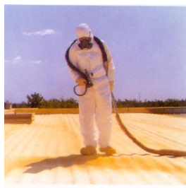
Spray for thermal insulation
